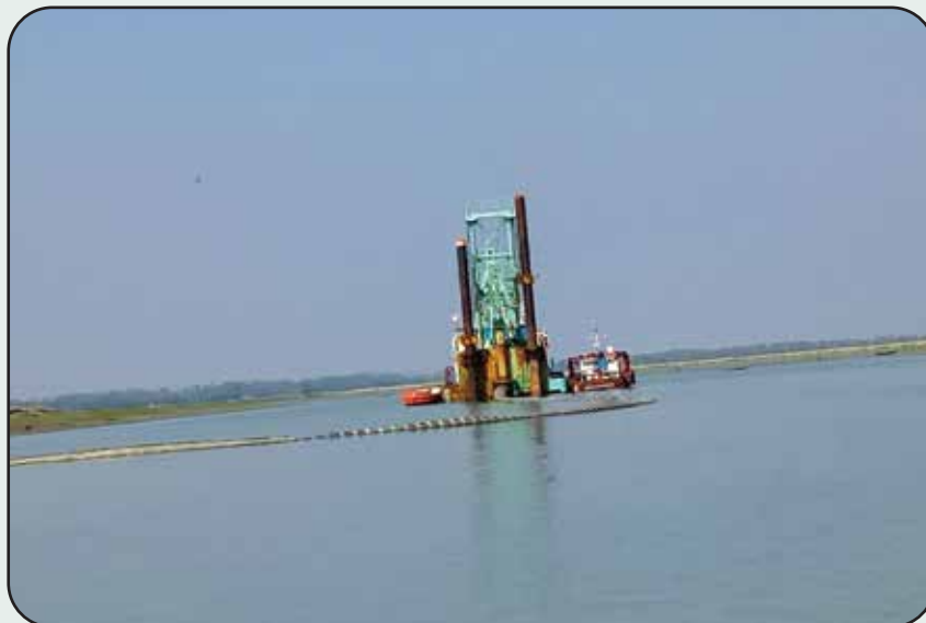
132/33 KV Sub-station Sand Filling Dredging Work
