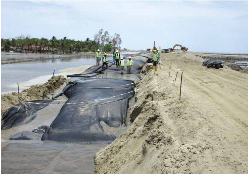
Protection of Dyke by geo-tube
